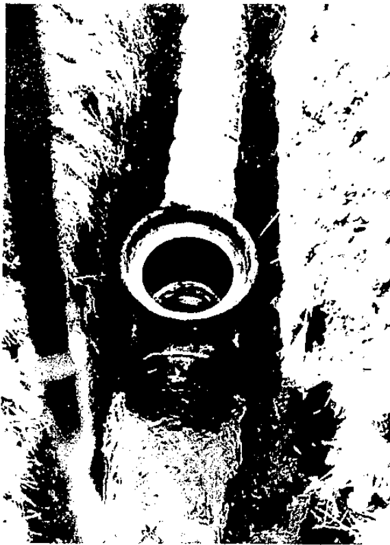
Fig. 12. Laying of lock.
