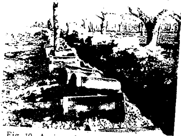
Fig. 10. A view of trenching of collecting canal.
